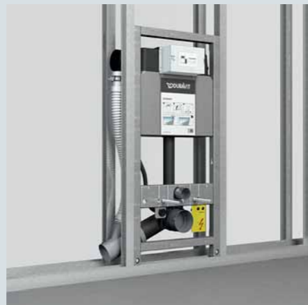
Dry-wall installation in a plasterboard wall frame
